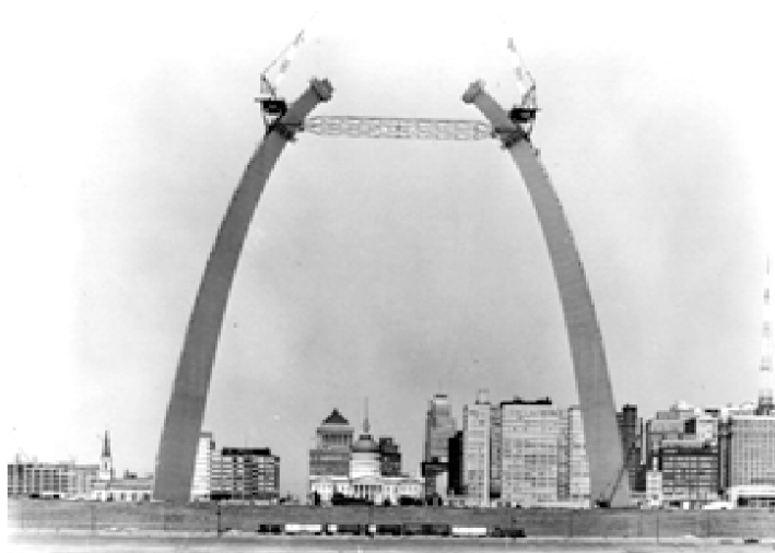
Figure 11 St. Louis gateway arch with sacrificial truss
